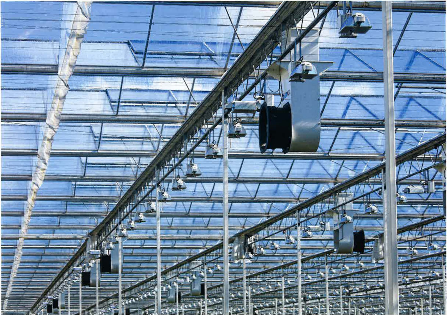
A new type of fan can mix dry and cold air from above a closed screen with greenhouse air. It enables dehumidification and heat removal.
